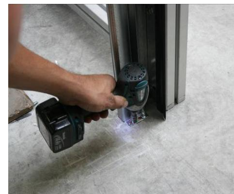
Manual for installing anti-burglar brackets in (garage) doors. View a demonstration movie on installation and on burglar attempts with and without the system on FlexiForce FF-TV channel on Youtube®
